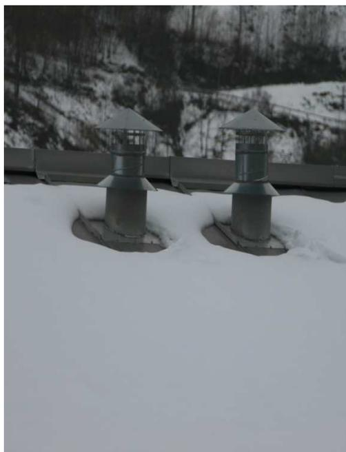
Intake in a flat or slightly slant roof-plane below or equal to an exhaust in the same or an adjacent part of the roof, also flat or slightly slant (maximum pitch < 23°).
