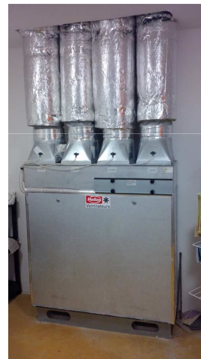
VMC double flux secondaire
