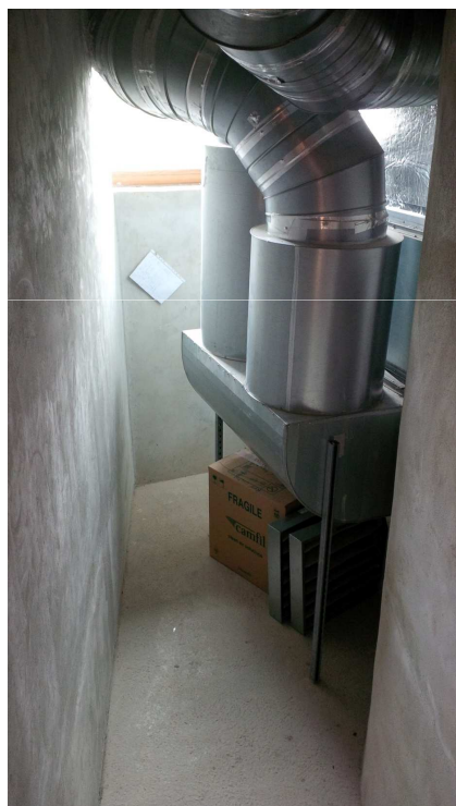
VMC double flux principale
